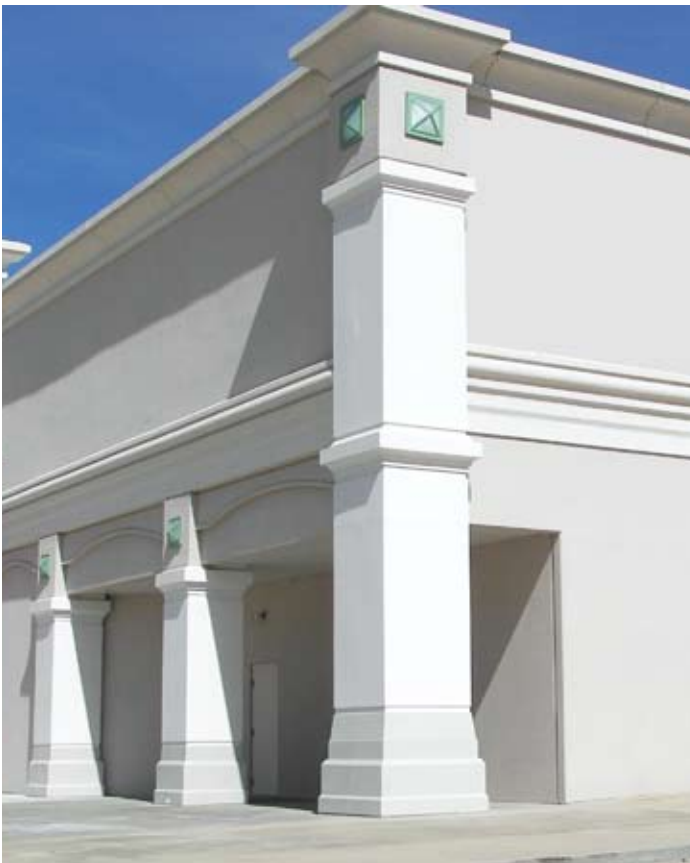
▼ Exterior Square Stacking Columns
