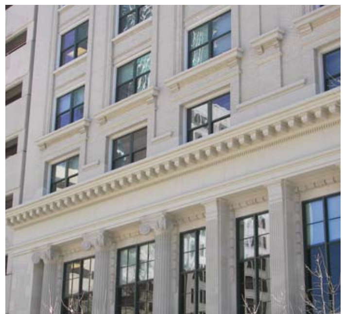
▼ Exterior Cornice Restoration
